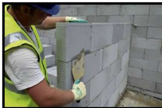
Fig. – 94 Thin Joint Masonry Technique
